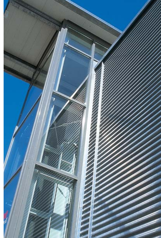
▲ Contractor: Sinhor - QUARTZ-ZINC®
